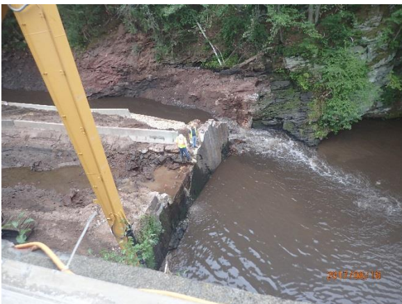
The dam is lowered and water diverted to one side.
