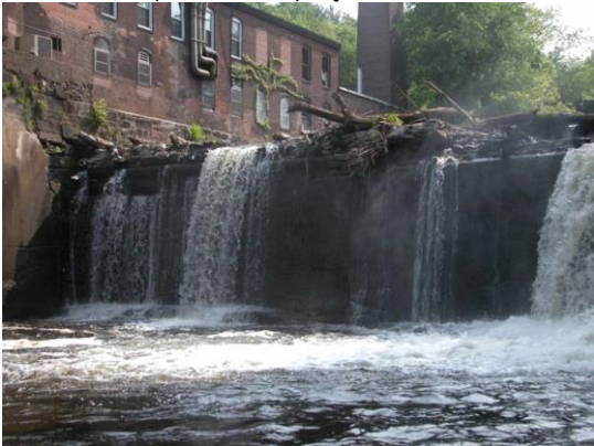
The Springborn Dam was over 20 feet high and a complete barrier to migratory fishes. The impoundment was full of contaminated sediment and debris.
